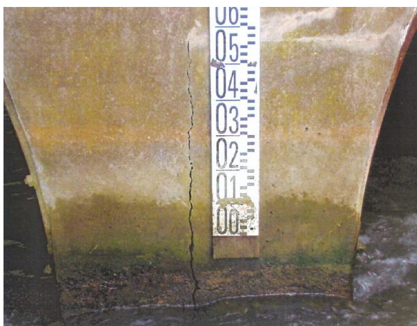
Fissuration verticale
